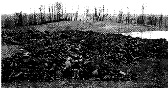
Mined area at Zeb Mountain planting site, previously covered with compacted soil according to traditional reclamation procedures, is being prepared with the Forestry Reclamation Approach method. The FRA method involves planting American chestnut seeds in loose, rocky soil.
