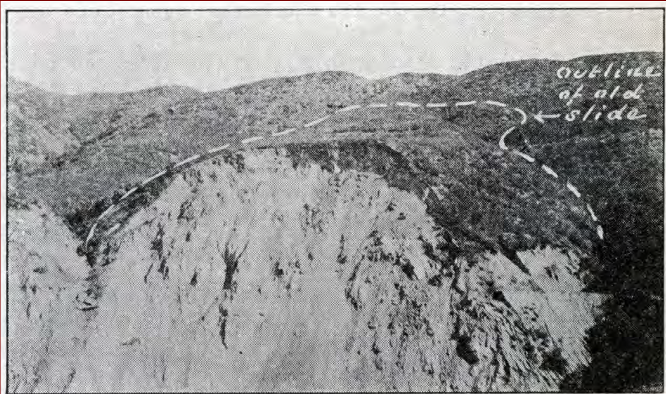
Fig. 8. East Abutment Showing Outline of Old Slide Above Present Slide
