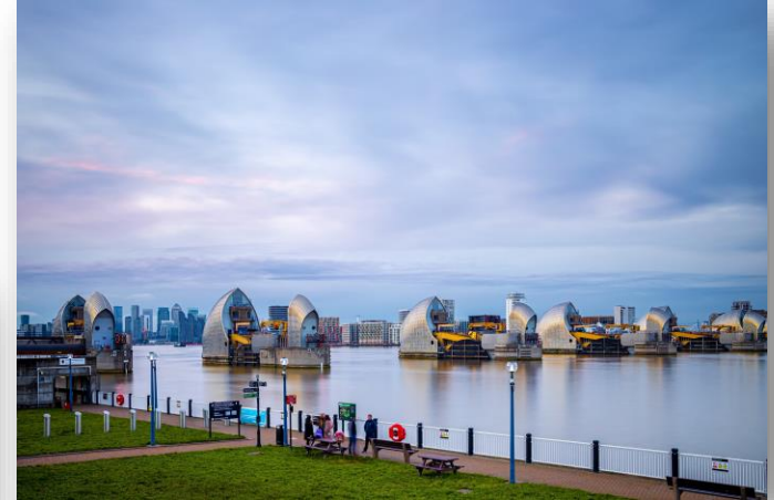
The Thames Barrier that protects the City of London from flooding due to storm surges, was designed with an annual exceedance probability (AEP) of 0.001, i.e., a 0.1% chance of flooding in any year.
