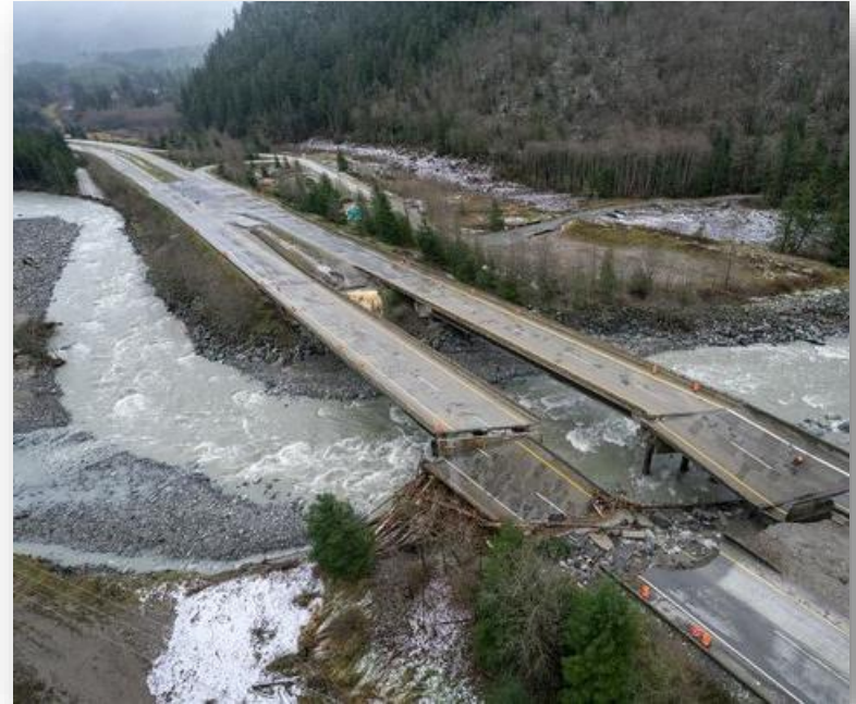
Roadways damaged by heavy rains and mudslides along the Coquihalla Highway near Hope, B.C, Canada Photo source: Jonathan Hayward/The Canadian Press
